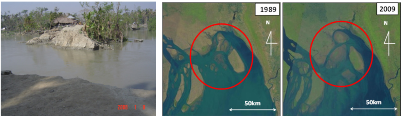
Figure 1. (a) Washed away embankment after cyclone Sidr in 2007, (b) and (c) show the satellite images of coastline changes at the north-eastern part of the Meghna Estuary
