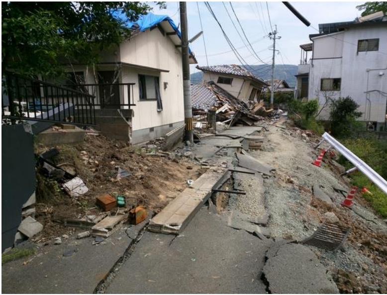
Many damaged roads
